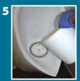
Insert new cartridge and fill with water.
