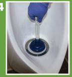
If the cartridge flow is slow or has stopped, you may extend the cartridge life by pouring water into the bowl and using a plunger to open the cartridge without removing it. It is recommended that the cartridge be replaced soon after using the plunger.
