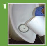
Pour water into the cartridge during routine cleaning, Dome removal recommended for this "flushing" of the system.
