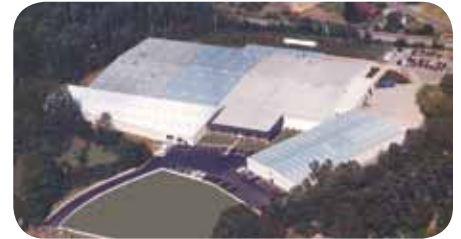
Corporate Headquarters and Nonwovens Manufacturing facility in Acworth, GA
